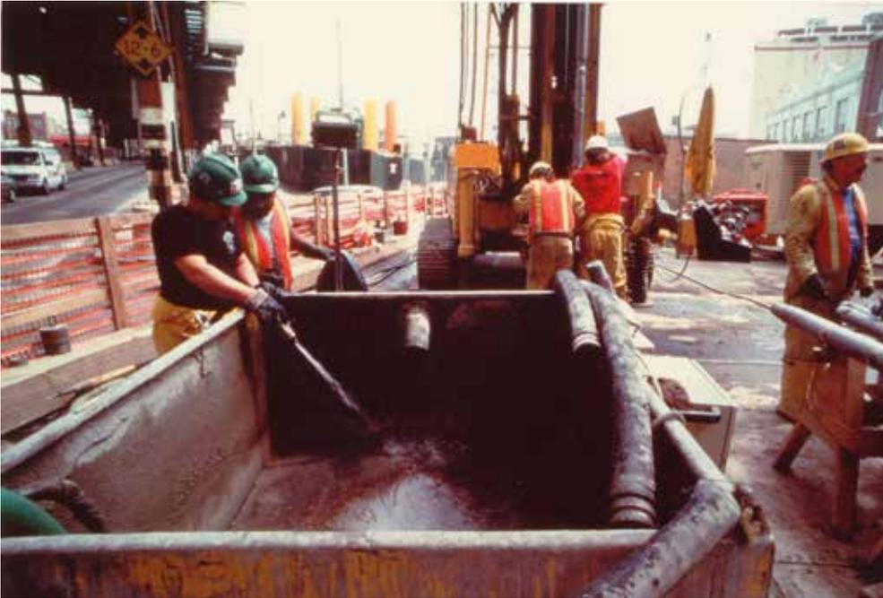
Fig. 6. Waste fluid collection tank.
